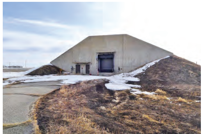
MSR warhead handling building exterior
